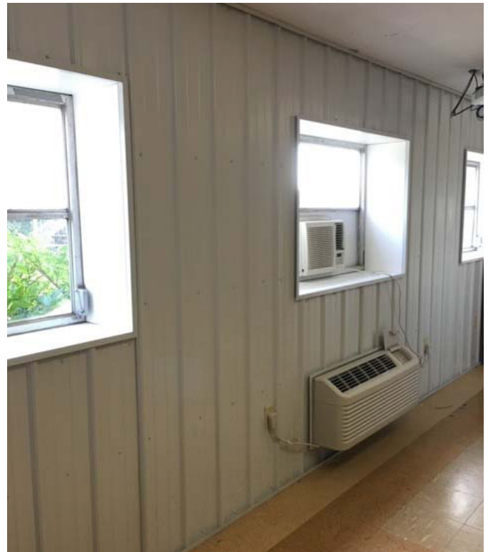
New classroom wall!
