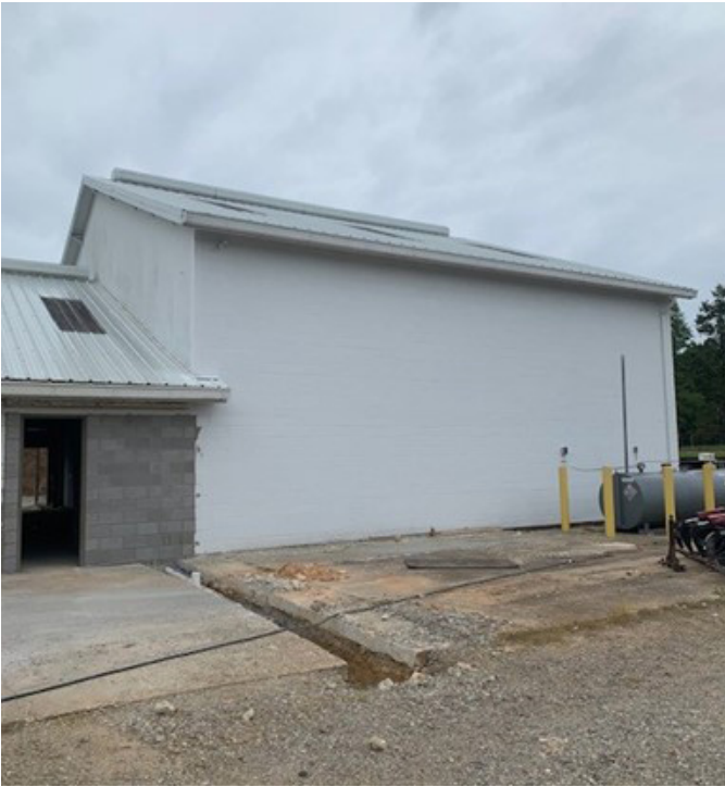
Converted Hay Storage Area
