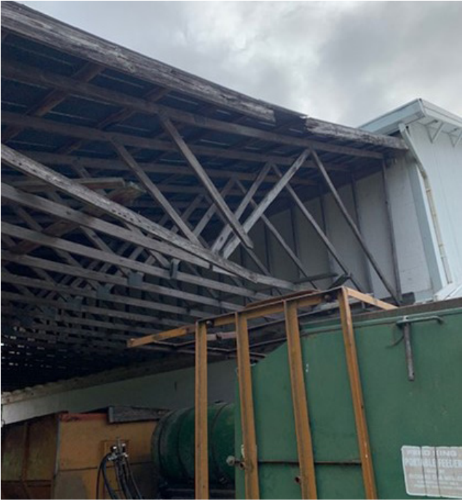
Equipment shed roof breaking on both ends
