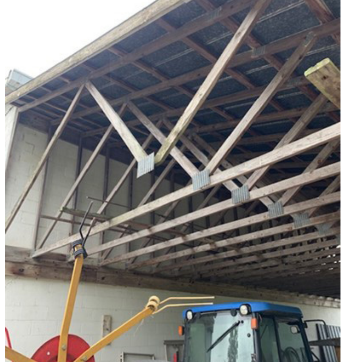
Equipment shed roof breaking on both ends
