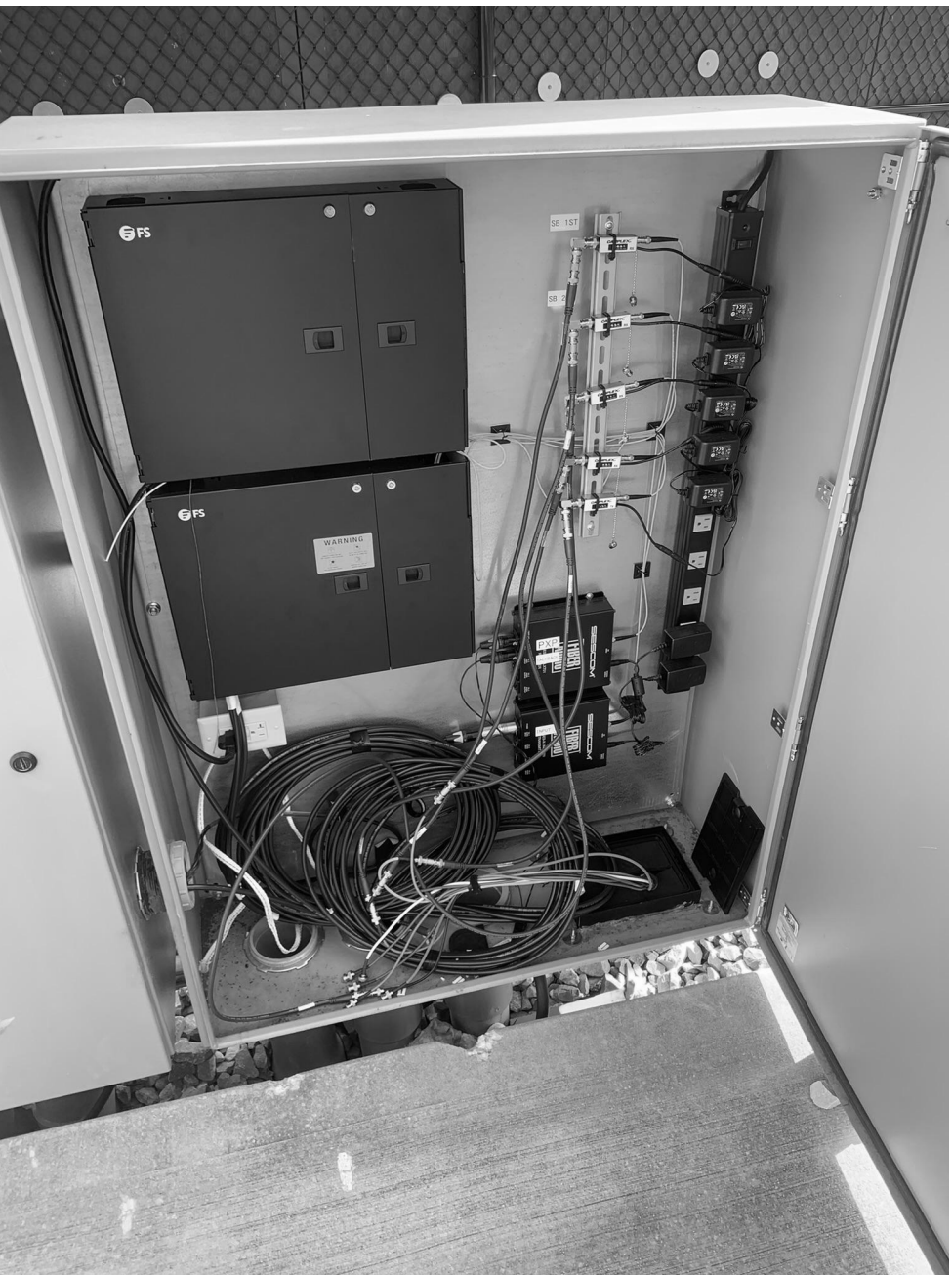
CAMERA TERMINATION BOX DETAIL NO SCALE
