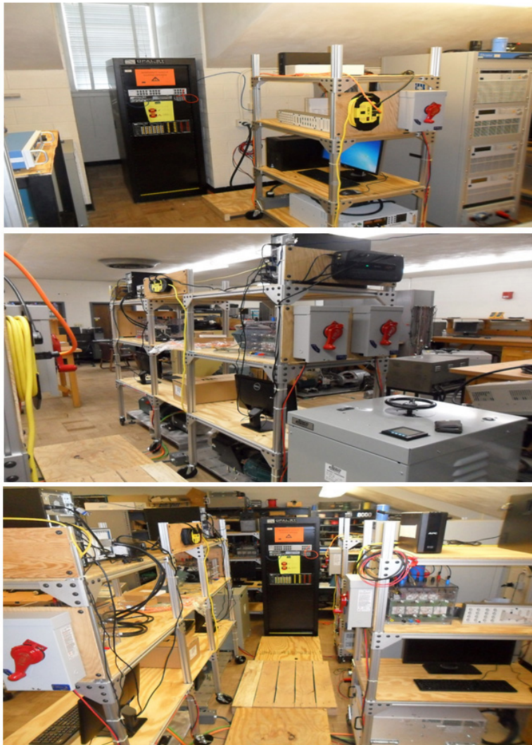
Dr. Joseph Ojo's DC-Bus Testbed Lab developed under the Durrig ONR Project
