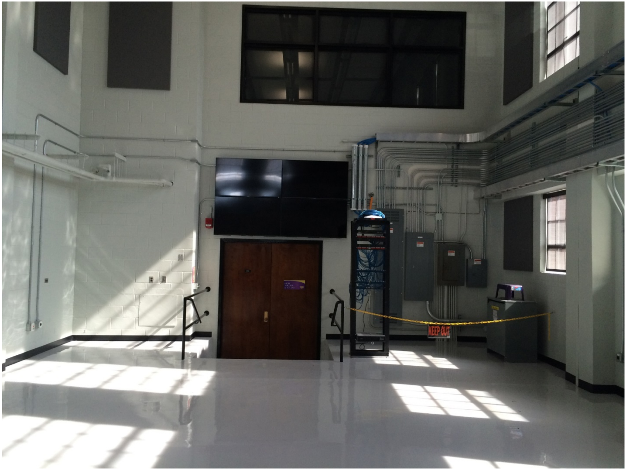
CESR—New Home of the SMART GRID LAB [Renovation just completed]
