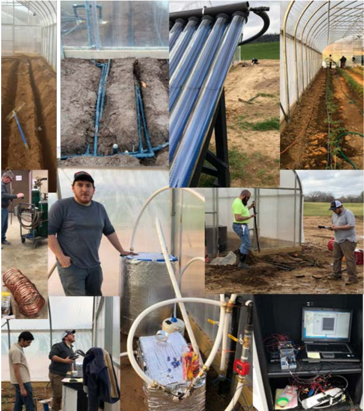
Undergraduate Aaron Bain, Graduate student Vinit Prabhu, Geothermal contractor Jason Gentry, and Ch.E. Technician Perry Milton working on various stages of a project to heat the roots of tomato plants using solar thermal energy.
